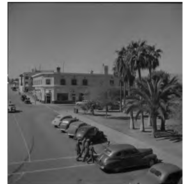
Figure 192 General view of a street leading to the depot of the Atchison, Topeka, and Santa Fe Railroad, Needles, CA; Library of Congress, Prints & Photographs Division, FSA/OWI Collection, [reproduction number, LC-USW3-021415-E]
